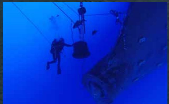
UNDERWATER REPAIRS - MID-ATLANTIC
