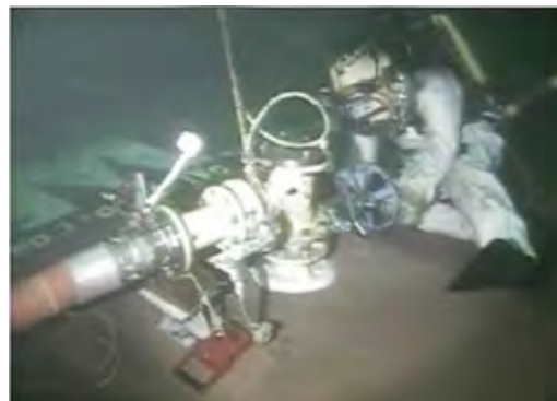
Salvage diver working to remove fuel from a sunken vessel
