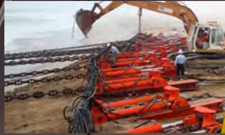
Using chain pullers and chain cutting
