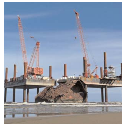
Titan Salvage began work in June to remove the stubborn remains of the New Carissa , in Coos Bay. Two jack-up barges, Karlissa A and Karlissa B , are working at the site. The vessel ran aground in February 1999. Earlier salvage attempts were dogged by difficulties. Due to the area's notoriously heavy swells, work platforms are essential for this operation.
